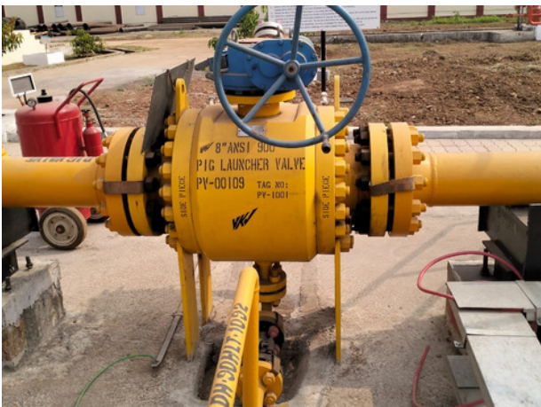
VKVC Site Photographs of Pig Launcher & Pig Receiver Valves.
