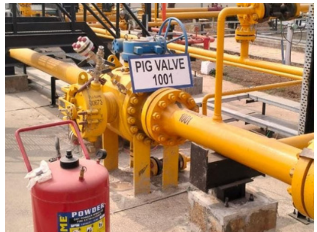
VKVC Site Photographs of Pig Launcher & Pig Receiver Valves.
